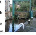
• When water levels have equalised, open the mitre door or guillotine gates fully to allow entry into the lock and follow the procedures outlines above for lock use.
